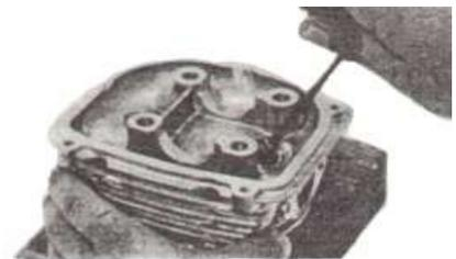
16. Measure valve guide inside diameter.
